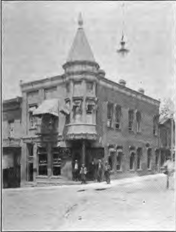
NATIONAL BANK OF SUMMERS, IN 1905, Cor. Temple Street and Third Avenue.
